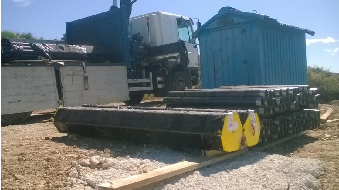
Figure 2: Drilling preparation for an incline geotechnical drill hole at Muga mine
